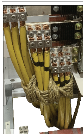
Figure 42 - Cable Restraint Examples
